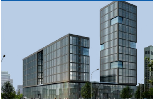
Parking Lot project in Dahua Hangzhou
