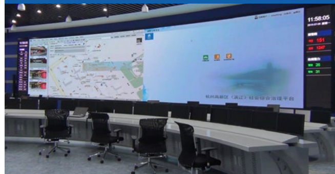
Hangzhou Traffic Command Center
